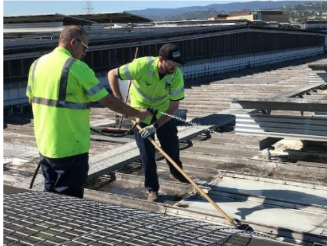
Cleaning TS and MRF Roof Skylights
