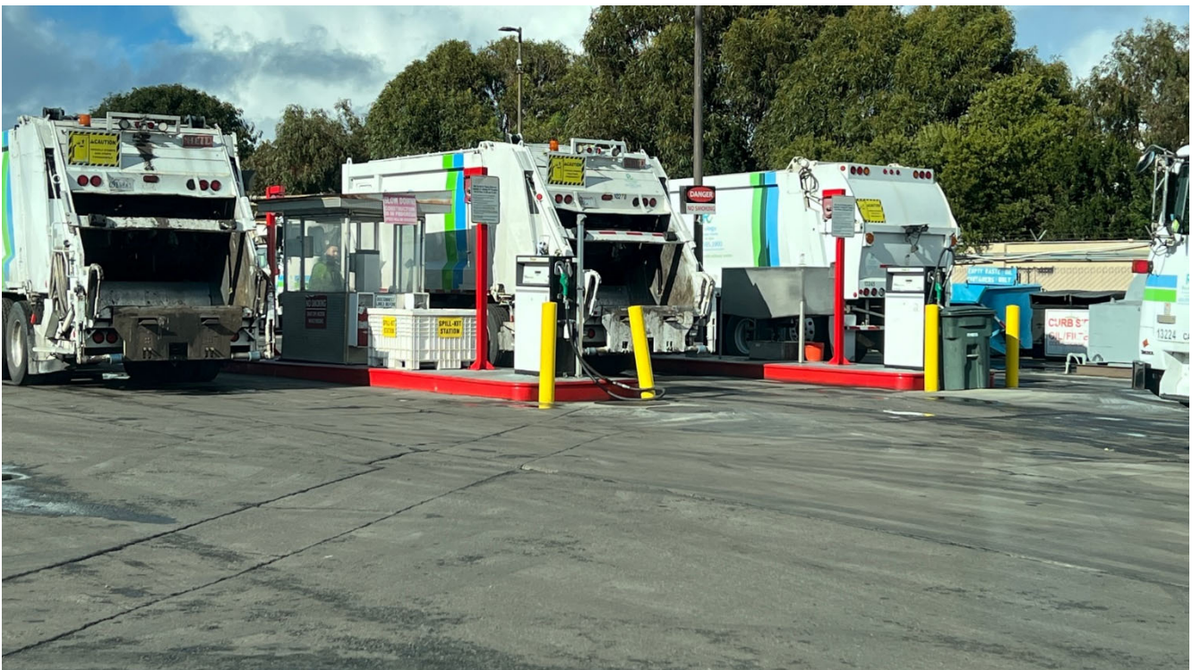
Figure 3 Truck Fueling at UST Station
