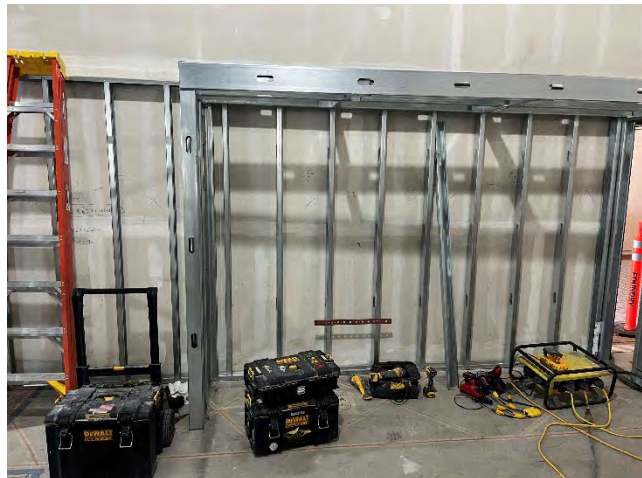
1st floor – Kitchenette built-in wall
