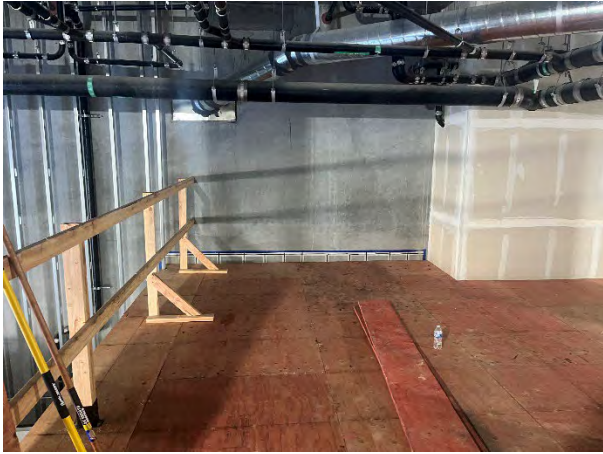
2nd floor - Deck looking at mini-conference room
