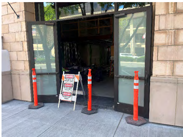
1st floor - exterior street front door into flex area
