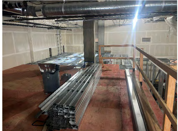
2nd floor - Deck
