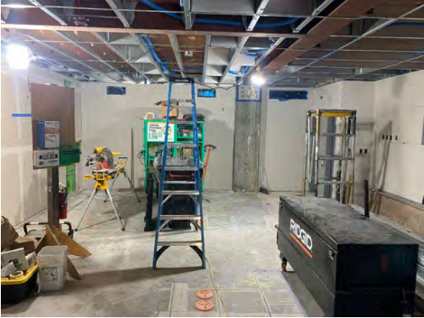
1st floor Inside main conference room
