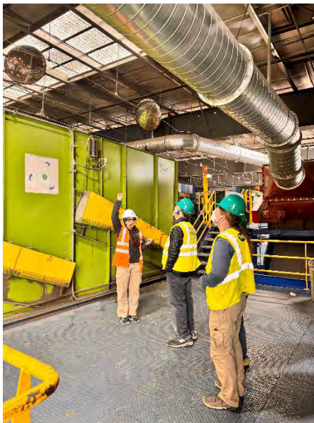
Public Outreach Fellow Manpreet Chandok leading a public tour in the Materials Recovery Facility at Shoreway.
